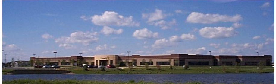
ONTRACK's corporate headquarters facility in Eden Prairie, MN.
